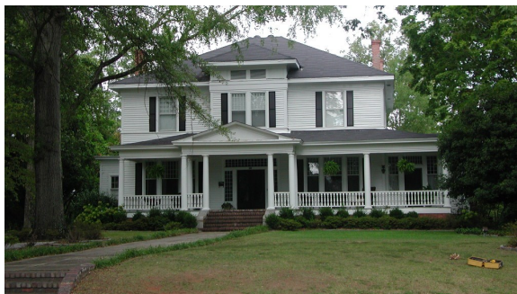
16 369 Heard Street Atlanta physician Dr. A.S. Hawes had this Classic Box style home built in 1905. After moving to Elberton, Hawes became a successful businessman.
