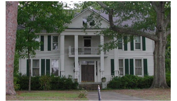
9 326 Heard Street The William Tustin Van Duzer House is among Elberton's oldest, built in the mid-1800's. It features Greek Revival architecture.
